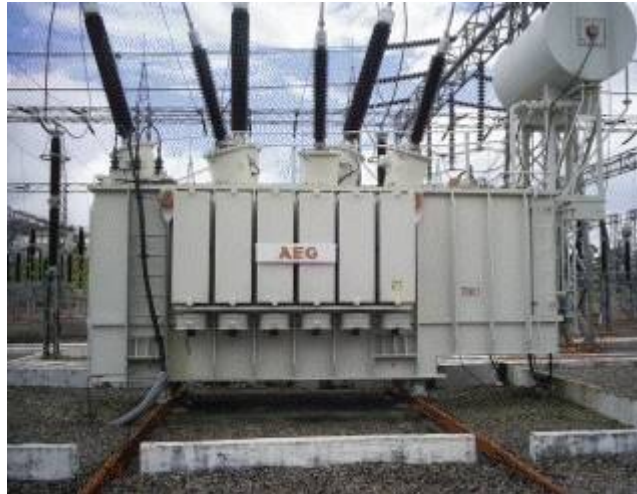
Figure II.3-2 Example 132/33 kV Oil Transformer, Courtesy of AEG
