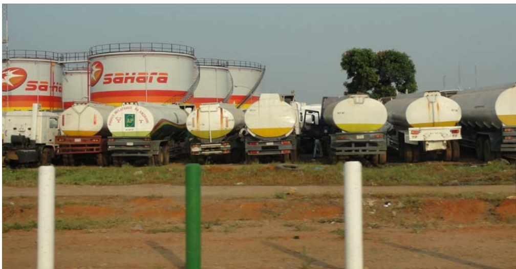
Figure II.6-4 Nigerian CTMV with fuel storage tanks
