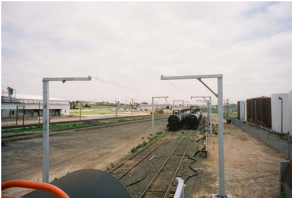
Figure II.6-8 Example design for train top loading facility (top), train bottom loading facility (bottom)
